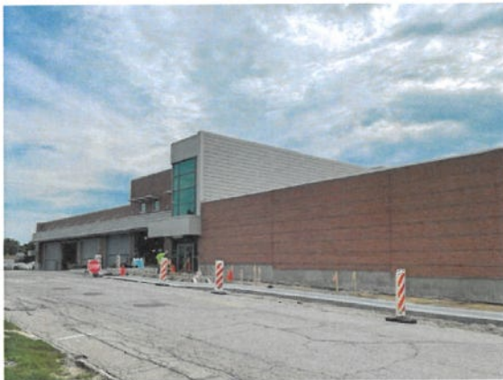
Figure 15: Construction Progress Photo 8-18-2026
