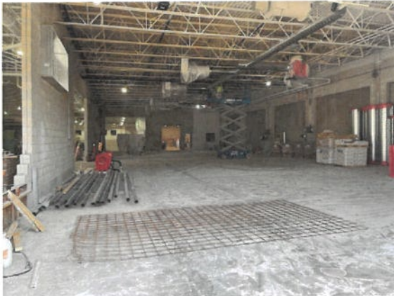
Figure 19: Construction Progress Photo 8-26-2026
