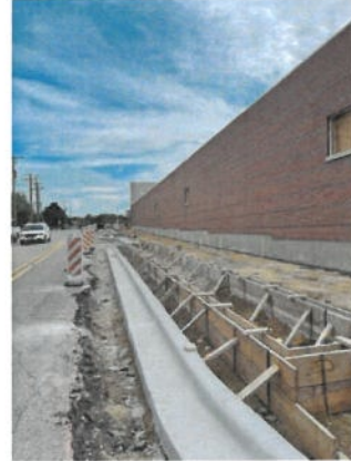
Figure 14: Construction Progress Photo 8-18-2026
