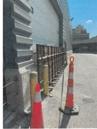
Figure 20: Construction Progress Photo 8-26-2026
