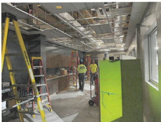
Figure 29: Construction Progress Photo 8-26-2026
