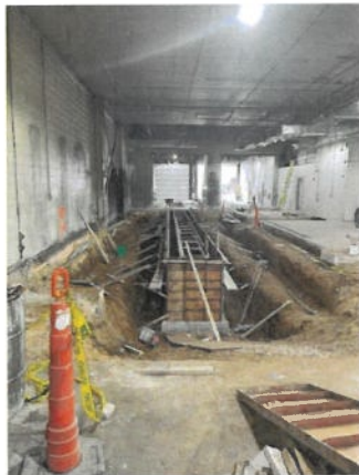
Figure 5: Construction Progress Photo 8-4-2026
