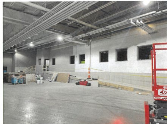
Figure 28: Construction Progress Photo 8-26-2026
