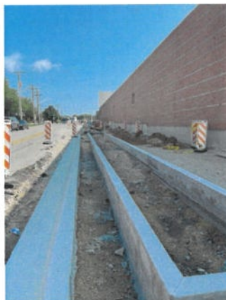
Figure 17: Construction Progress Photo 8-26-2026
