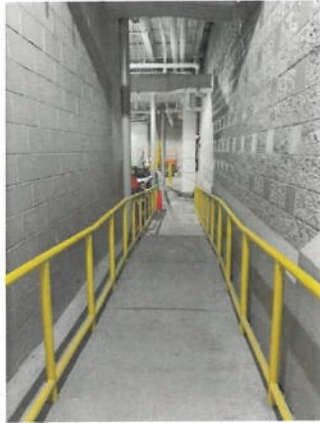
Figure 31: Construction Progress Photo 8-26-2026
