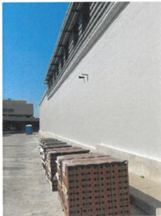
Figure 21: Construction Progress Photo 8-26-2026
