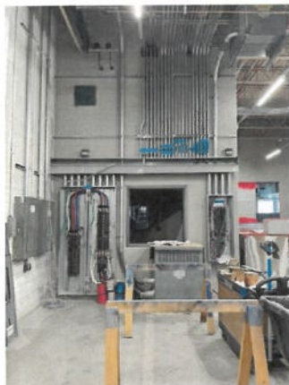
Figure 27: Construction Progress Photo 8-26-2026
