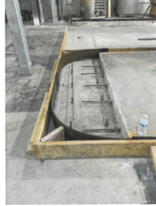
Figure 34: Construction Progress Photo 8-26-2026
