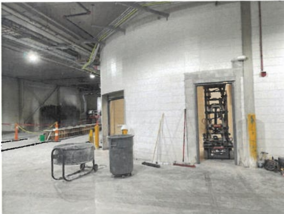
Figure 33: Construction Progress Photo 8-26-2026
