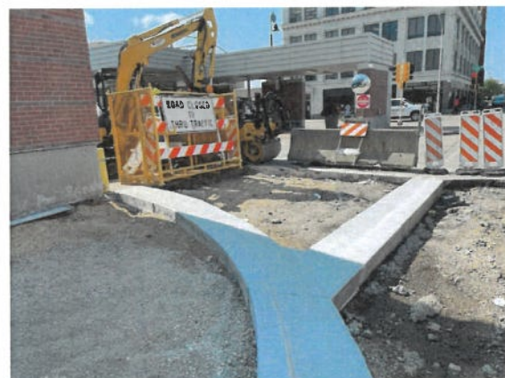
Figure 18: Construction Progress Photo 8-26-2026
