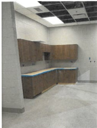
Figure 25: Construction Progress Photo 8-26-2026
