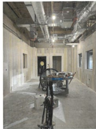
Figure 10: Construction Progress Photo 8-4-2026
