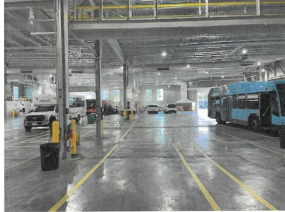
Figure 32: Construction Progress Photo 8-26-2026
