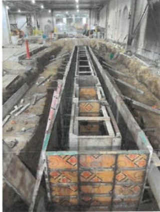
Figure 7: Construction Progress Photo 8-4-2026
