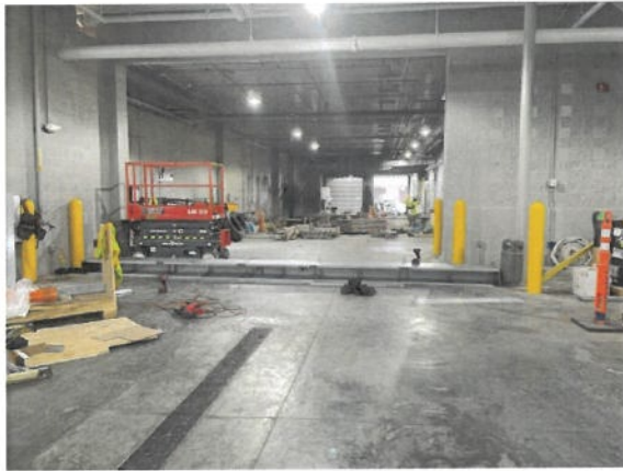
Figure 3: Construction Progress Photo 8-4-2026
