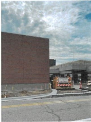
Figure 13: Construction Progress Photo 8-18-2026
