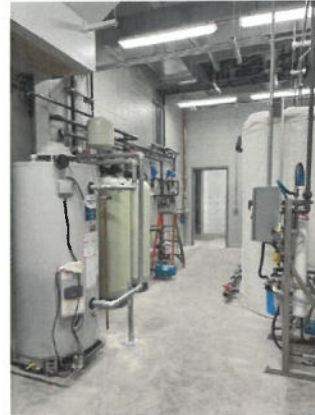
Figure 26: Construction Progress Photo 8-26-2026
