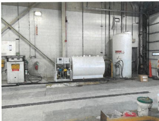
Figure 35: Construction Progress Photo 8-26-2026
