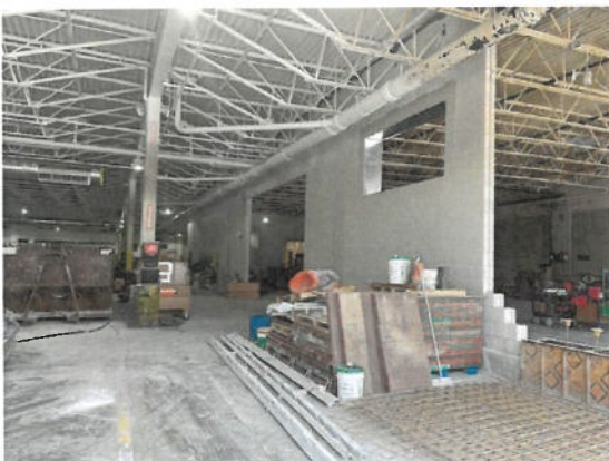
Figure 11: Construction Progress Photo 8-4-2026
