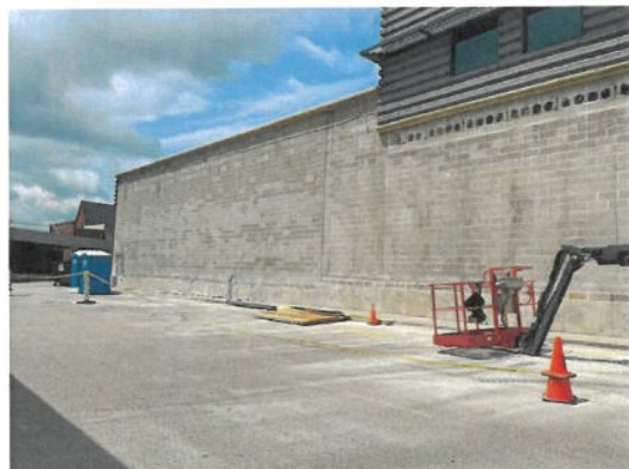
Figure 12: Construction Progress Photo 8-4-2026
