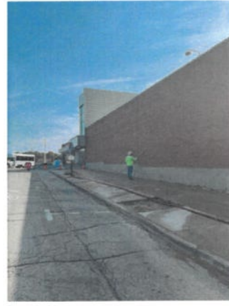
Figure 2: Construction Progress Photo 8-4-2026
