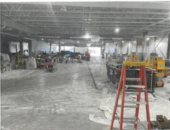
Figure 9: Construction Progress Photo 8-4-2026
