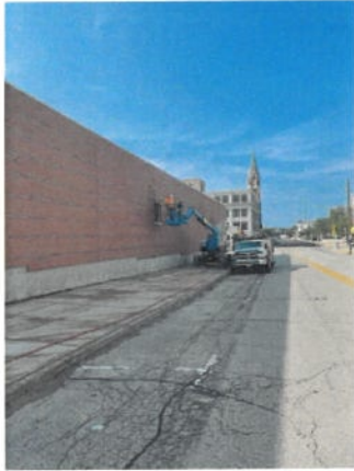
Figure 1: Construction Progress Photo 8-4-2026
