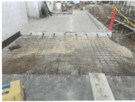
Figure 6: Construction Progress Photo 8-4-2026
