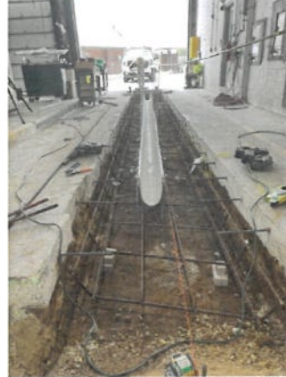
Figure 8: Construction Progress Photo 8-4-2026
