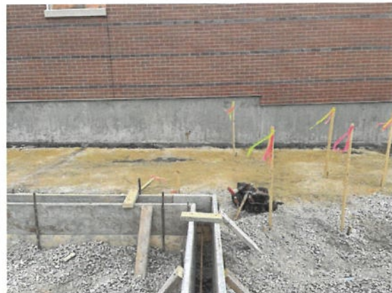
Figure 16: Construction Progress Photo 8-18-2026
