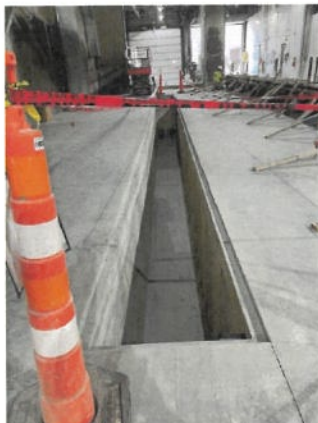
Figure 23: Construction Progress Photo 8-26-2026
