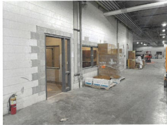
Figure 24: Construction Progress Photo 8-26-2026
