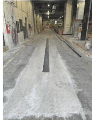
Figure 22: Construction Progress Photo 8-26-2026
