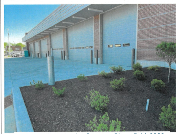
Figure 17: Construction Progress Photo 5-11-2026
