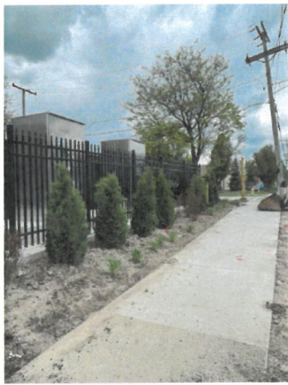
Figure 1: Construction Progress Photo 5-7-2026
