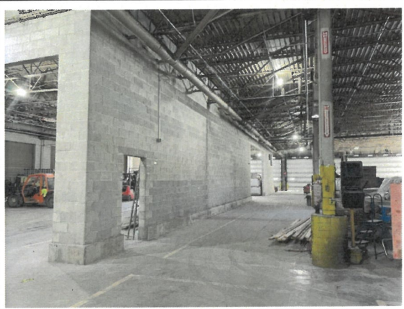
Figure 14: Construction Progress Photo 5-7-2026
