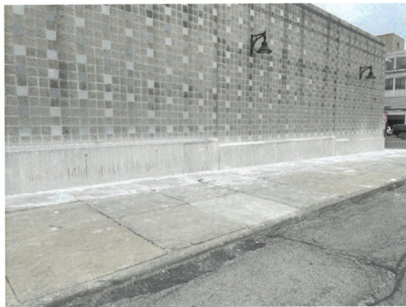
Figure 29: Construction Progress Photo 5-12-2026
