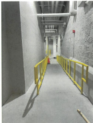
Figure 5: Construction Progress Photo 5-7-2026
