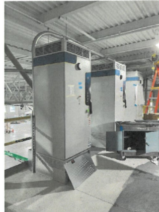
Figure 8: Construction Progress Photo 5-7-2026
