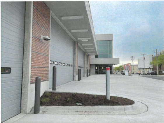
Figure 21: Construction Progress Photo 5-12-2026
