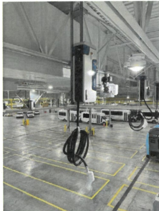
Figure 9: Construction Progress Photo 5-7-2026
