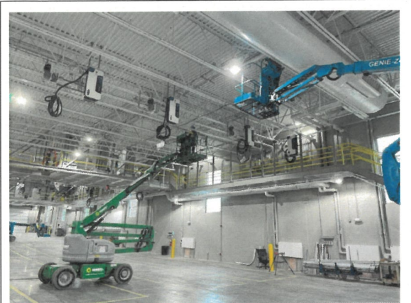
Figure 7: Construction Progress Photo 5-7-2026
