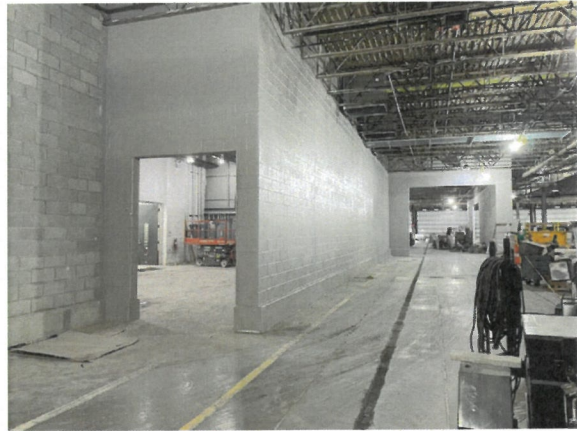
Figure 28: Construction Progress Photo 5-12-2026
