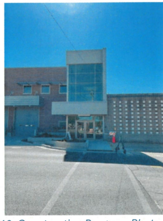
Figure 16: Construction Progress Photo 5-11-2026
