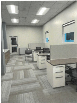
Figure 19: Construction Progress Photo 5-11-2026
