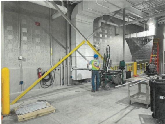
Figure 24: Construction Progress Photo 5-12-2026
