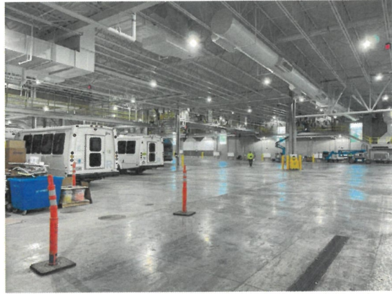
Figure 20: Construction Progress Photo 5-11-2026
