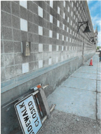
Figure 31: Construction Progress Photo 5-26-2026
