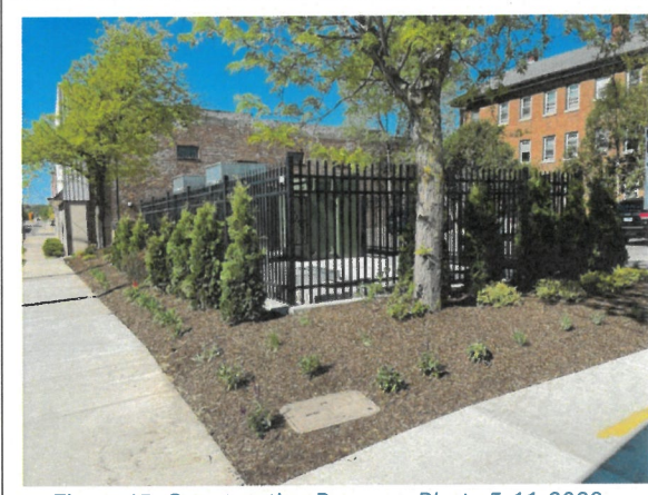
Figure 15: Construction Progress Photo 5-11-2026
