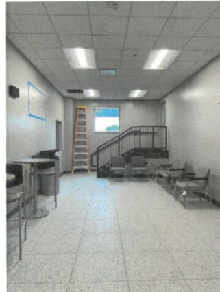
Figure 4: Construction Progress Photo 5-7-2026
