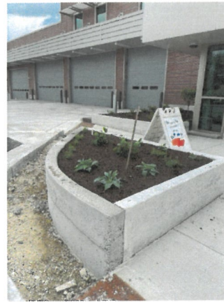
Figure 2: Construction Progress Photo 5-7-2026
