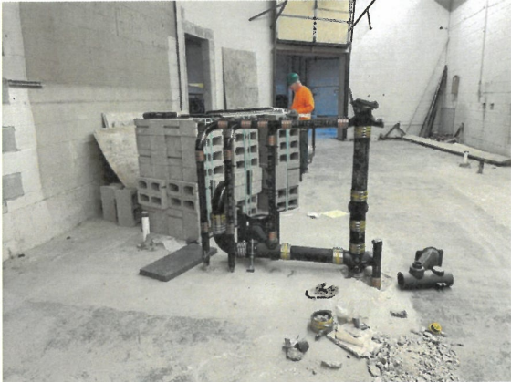
Figure 25: Construction Progress Photo 5-12-2026
