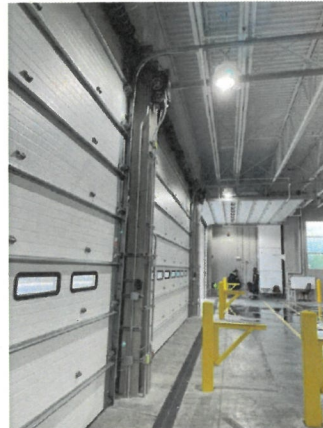
Figure 22: Construction Progress Photo 5-12-2026
