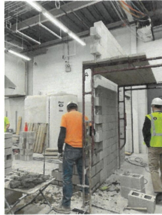
Figure 26: Construction Progress Photo 5-12-2026
