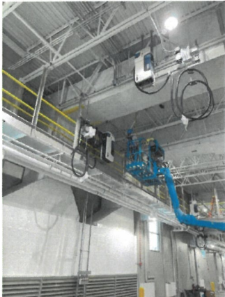
Figure 34: Construction Progress Photo 5-26-2026
