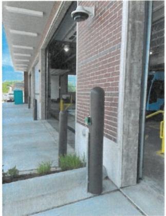
Figure 33: Construction Progress Photo 5-26-2026
