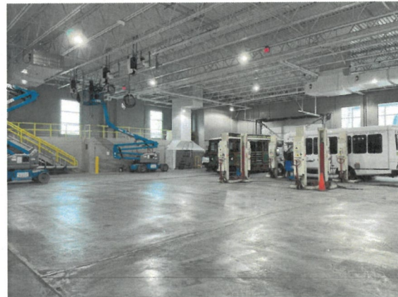
Figure 6: Construction Progress Photo 5-7-2026
