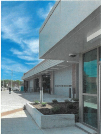
Figure 32: Construction Progress Photo 5-26-2026
