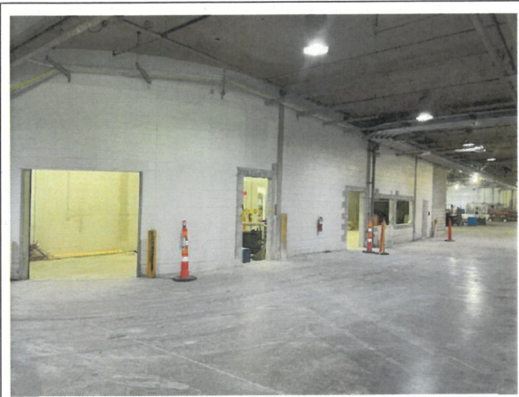
Figure 13: Construction Progress Photo 5-7-2026
