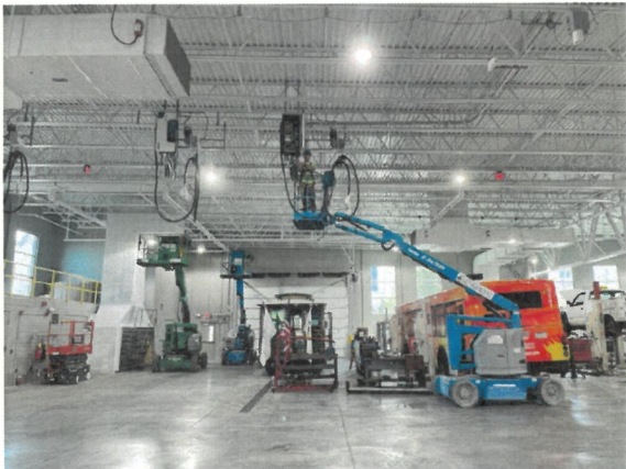
Figure 35: Construction Progress Photo 5-26-2026
