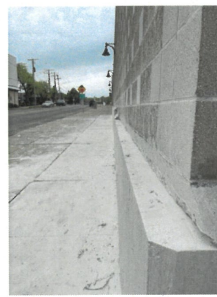
Figure 30: Construction Progress Photo 5-12-2026
