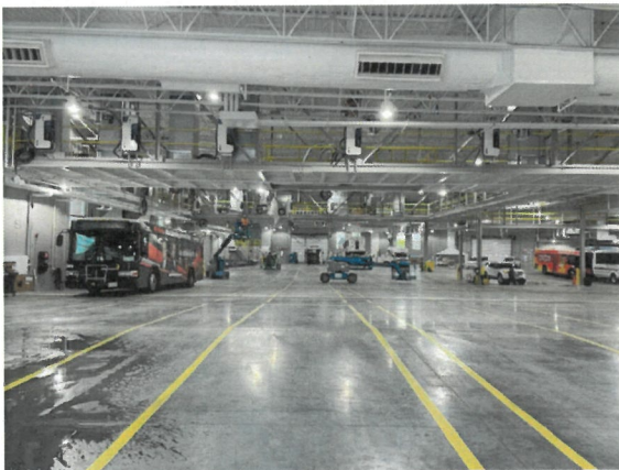
Figure 23: Construction Progress Photo 5-12-2026
