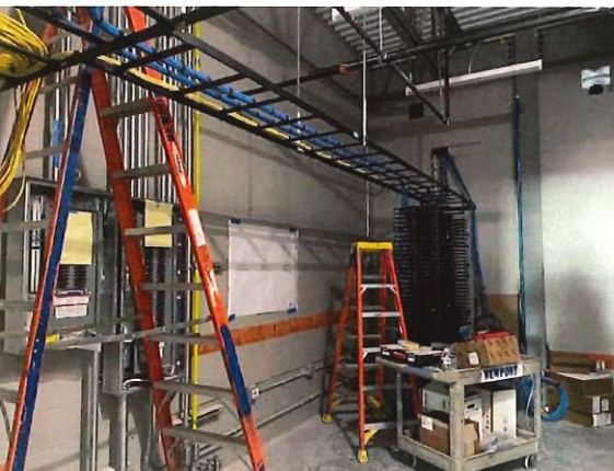
Figure 11: Construction Progress Photo 2-13-2026
