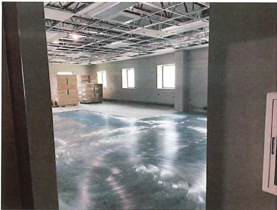
Figure 27: Construction Progress Photo 2-24-2026
