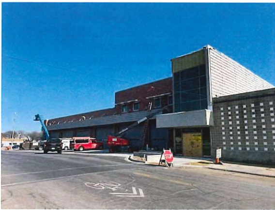
Figure 1: Construction Progress Photo 2-13-2026
