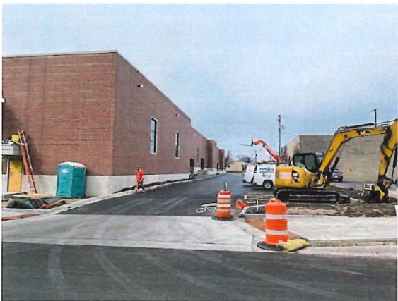
Figure 21: Construction Progress Photo 2-17-2026
