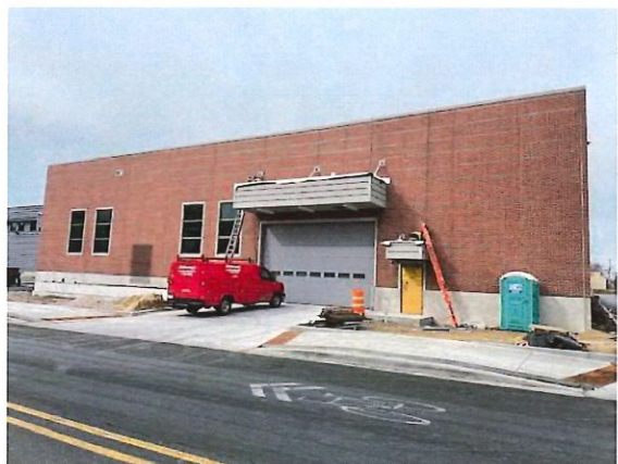
Figure 20: Construction Progress Photo 2-17-2026
