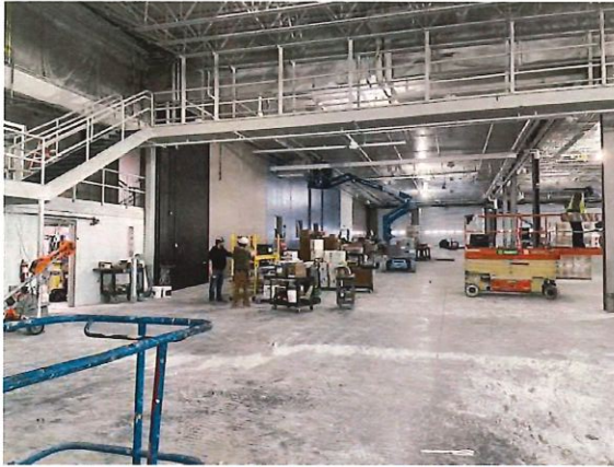
Figure 7: Construction Progress Photo 2-13-2026
