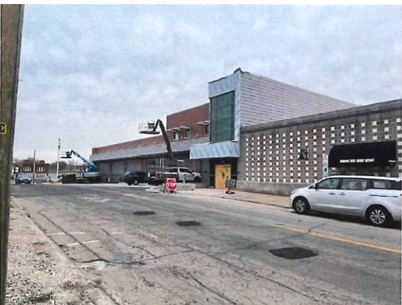
Figure 23: Construction Progress Photo 2-24-2026
