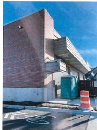
Figure 40: Construction Progress Photo 2-27-2026
