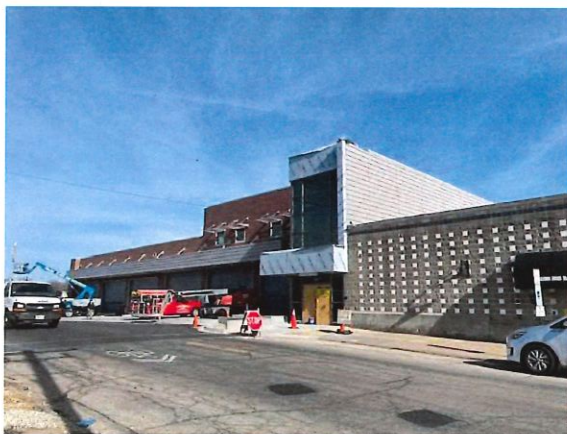
Figure 29: Construction Progress Photo 2-27-2026
