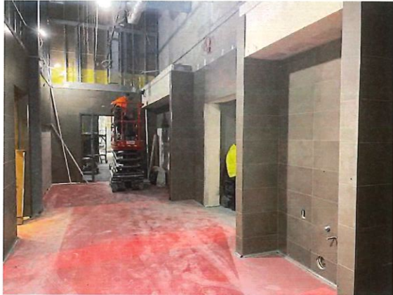
Figure 25: Construction Progress Photo 2-24-2026
