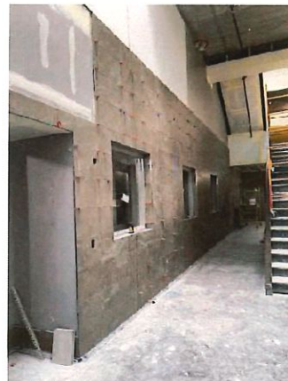
Figure 32: Construction Progress Photo 2-27-2026
