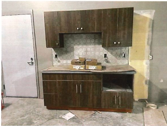
Figure 33: Construction Progress Photo 2-27-2026
