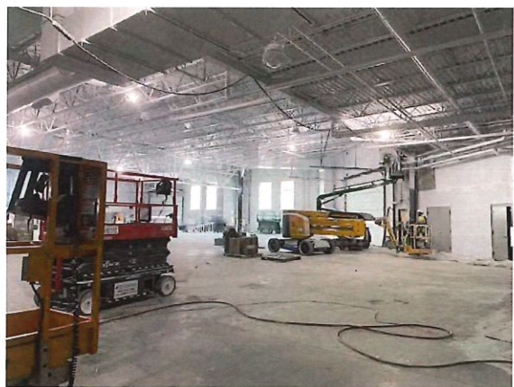
Figure 6: Construction Progress Photo 2-13-2026
