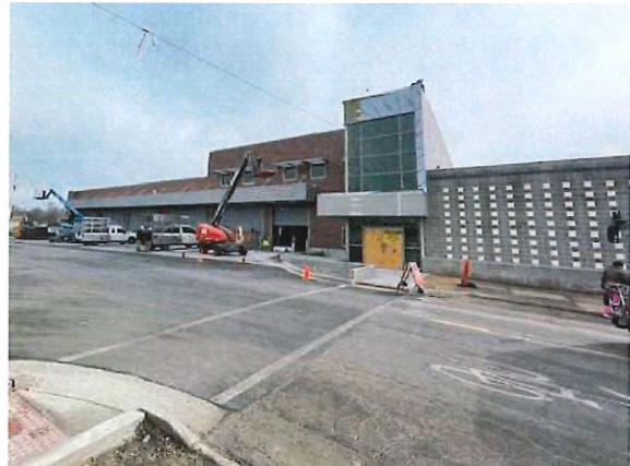
Figure 16: Construction Progress Photo 2-17-2026
