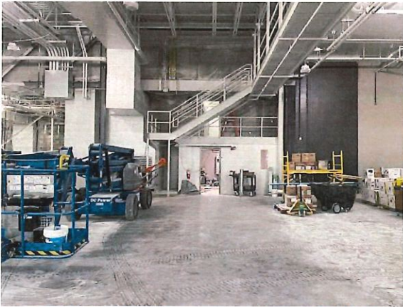
Figure 13: Construction Progress Photo 2-13-2026
