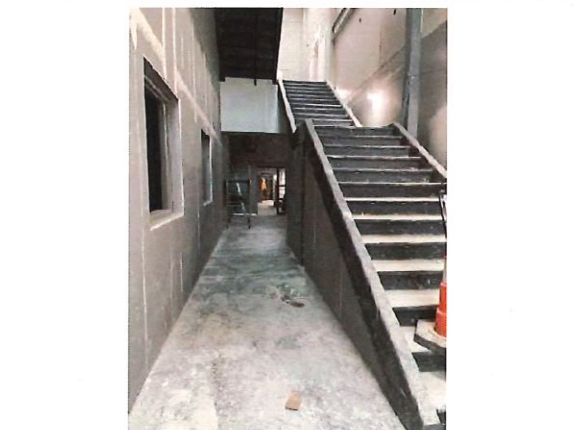
Figure 12: Construction Progress Photo 2-13-2026
