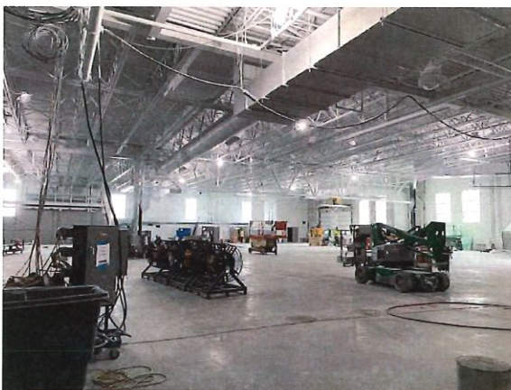
Figure 17: Construction Progress Photo 2-17-2026
