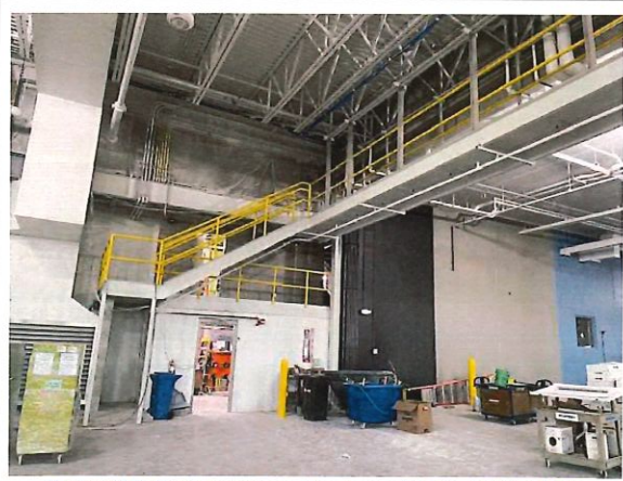
Figure 37: Construction Progress Photo 2-27-2026
