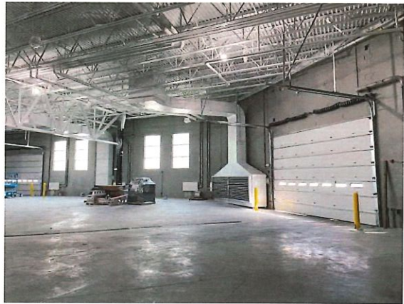
Figure 38: Construction Progress Photo 2-27-2026
