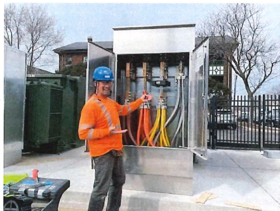
Figure 15: Construction Progress Photo 2-17-2026
