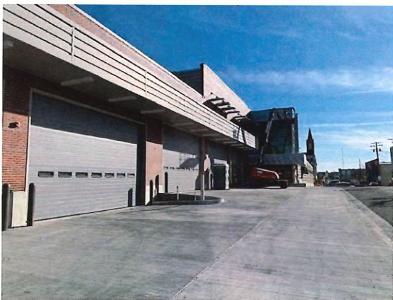
Figure 41: Construction Progress Photo 2-27-2026
