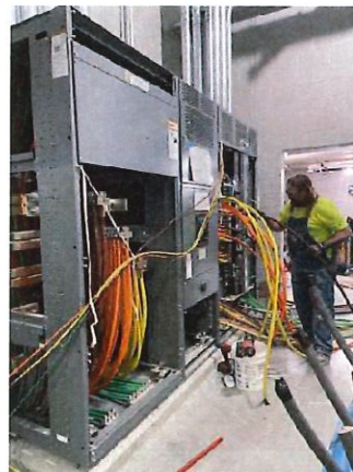
Figure 18: Construction Progress Photo 2-17-2026
