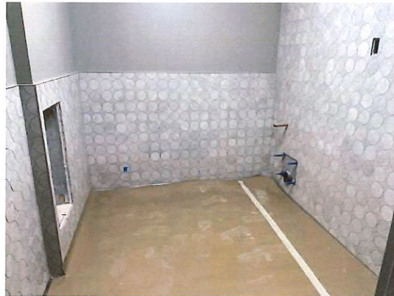
Figure 4: Construction Progress Photo 2-13-2026
