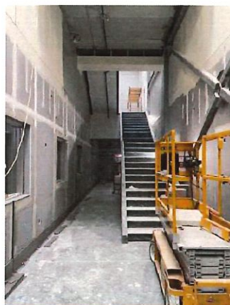
Figure 24: Construction Progress Photo 2-24-2026
