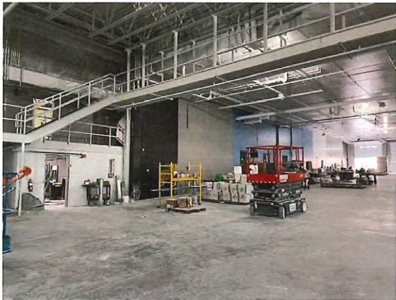
Figure 19: Construction Progress Photo 2-17-2026
