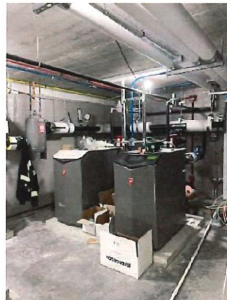
Figure 22: Construction Progress Photo 2-17-2026
