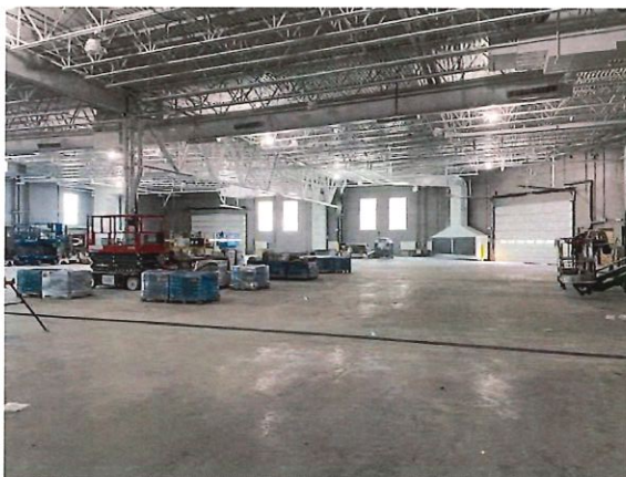
Figure 35: Construction Progress Photo 2-27-2026
