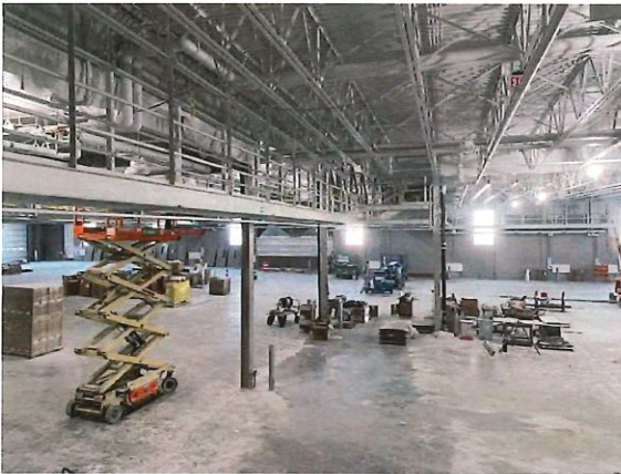
Figure 9: Construction Progress Photo 2-13-2026
