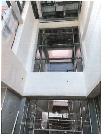
Figure 31: Construction Progress Photo 2-27-2026
