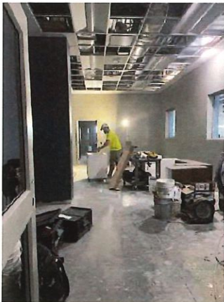
Figure 5: Construction Progress Photo 2-13-2026
