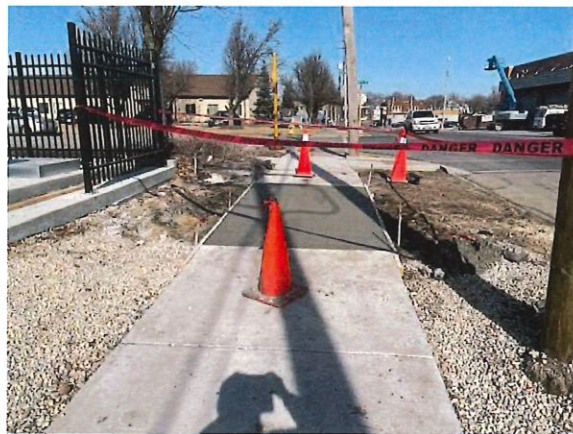
Figure 2: Construction Progress Photo 2-13-2026
