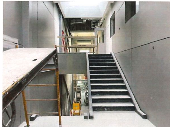
Figure 28: Construction Progress Photo 2-24-2026
