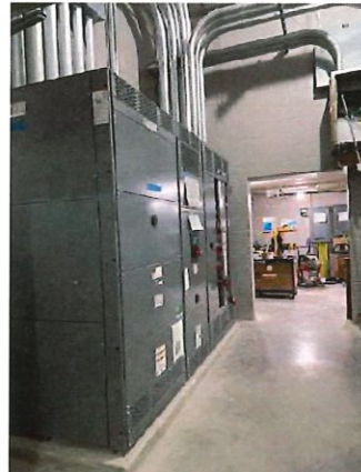
Figure 34: Construction Progress Photo 2-27-2026
