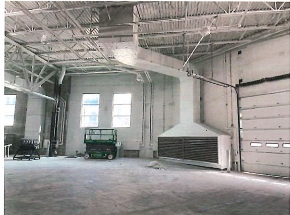
Figure 8: Construction Progress Photo 2-13-2026
