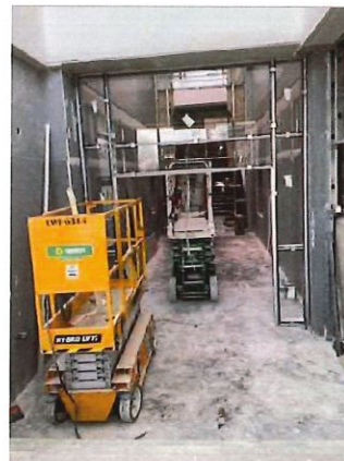
Figure 30: Construction Progress Photo 2-27-2026
