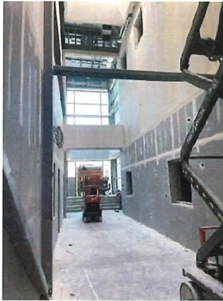
Figure 3: Construction Progress Photo 2-13-2026
