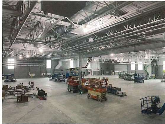
Figure 26: Construction Progress Photo 2-24-2026
