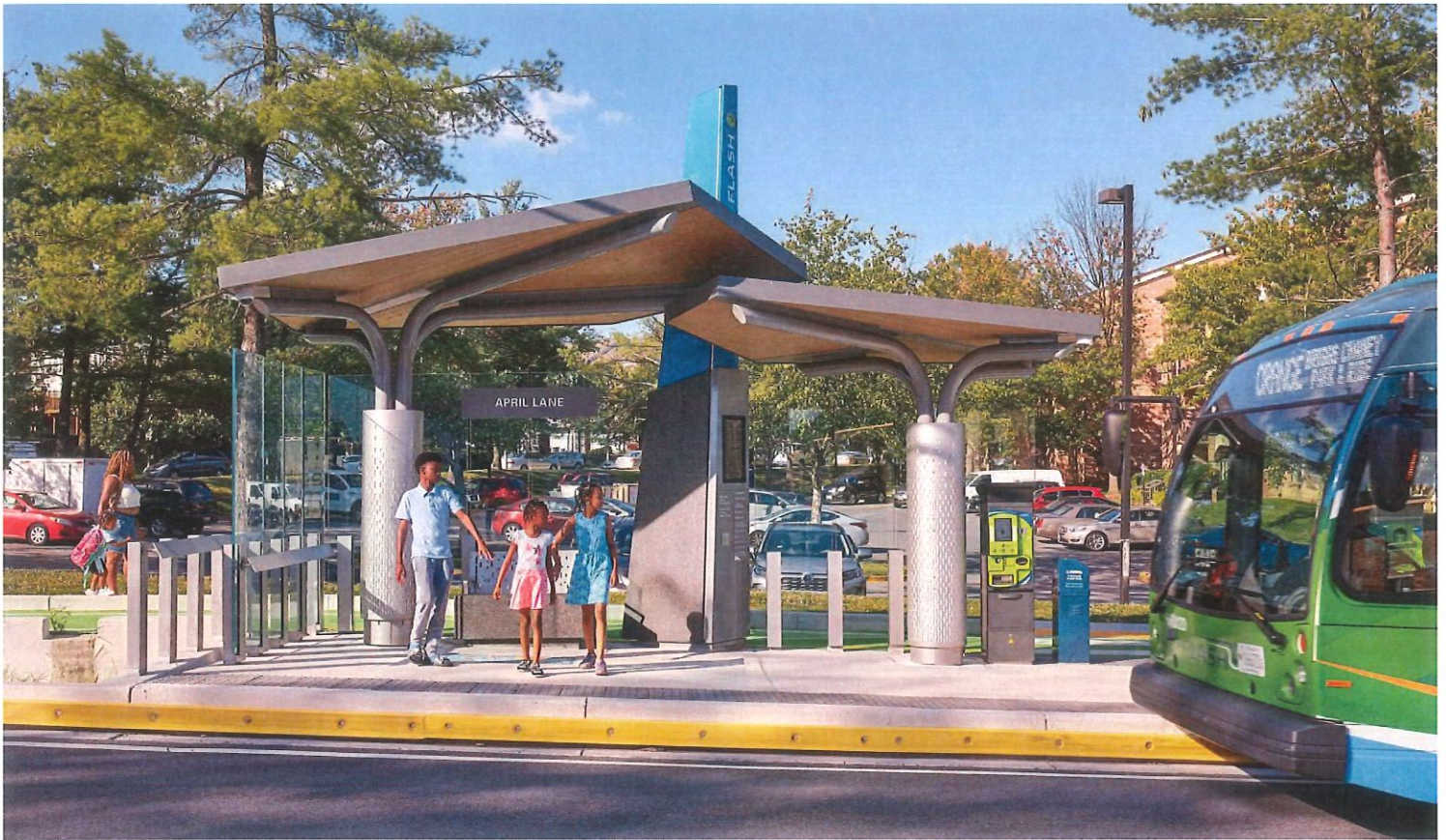
Figure 1. A rendering of a BRT station in Montgomery County, MD, featuring a vertical marker, real-time information, ticket vending machine, and near-level boarding. Source: ZGF.com
